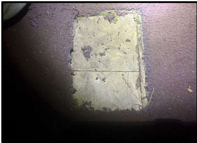
Photo #: 9 Material #: 9 Non-ACM Subject: View of white 9"x9" VCT, located in FS-1.
