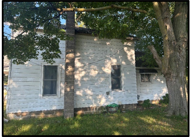
View of the property from the east.
