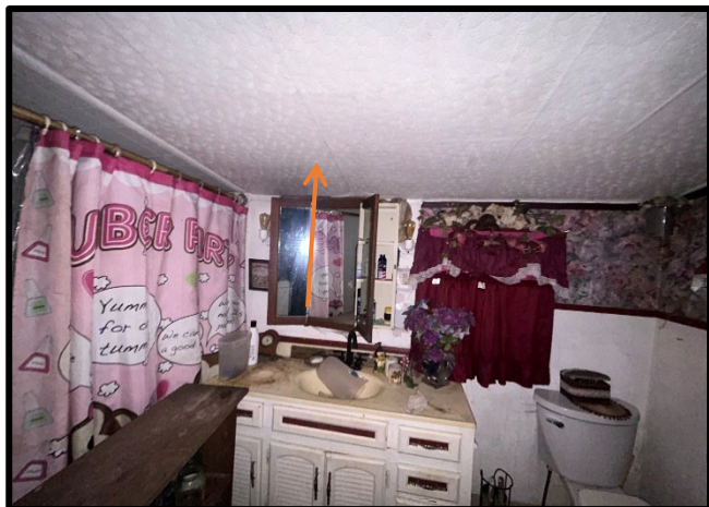
Photo #: 13 Material #: 13 Non-ACM Subject: View of shell pattern ceiling covering, located in FS-1.
