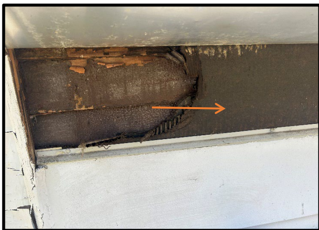
Photo #: 17 Material #: 17 Non-ACM Subject: View of black corrugated exterior wall vapor barrier, located in FS-3.
