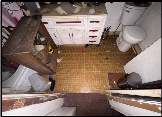
Photo #: 7 Material #: 7 Non-ACM Subject: View of yellow square pattern VSF, located in FS-1.
