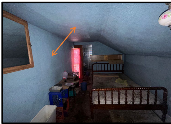
Photo #: 11 Material #: 11 Non-ACM Subject: View of rolled on wall and ceiling texture, located in FS-2.
